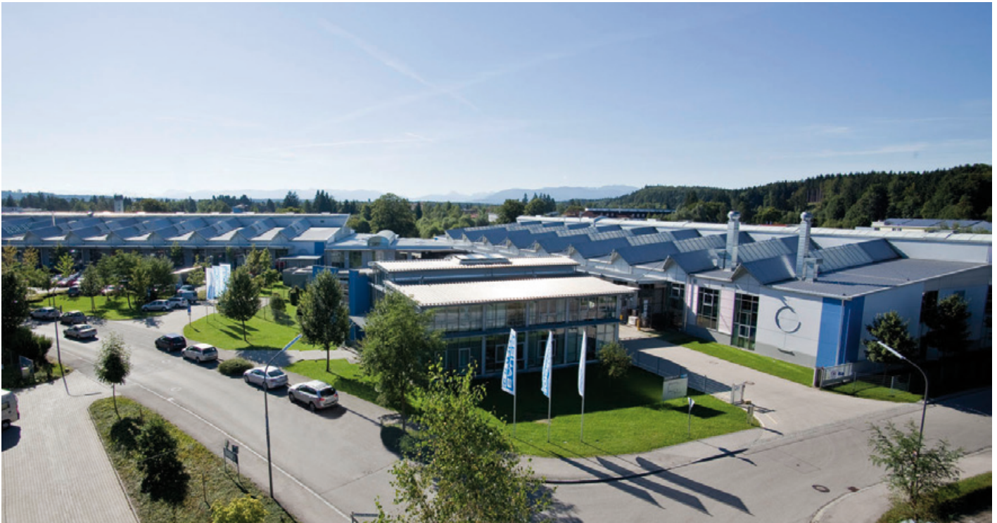
BAUER KOMPRESSOREN Plant I – Geretsried, Germany
